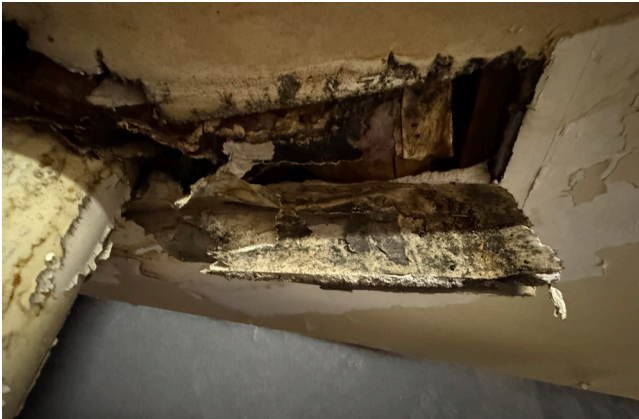
Drywall damage and some partial repairs from prior roof leaks.
