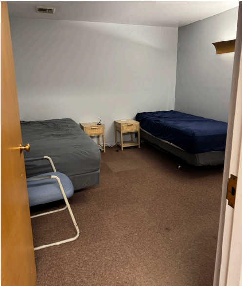
Egress path through sleeping room.
