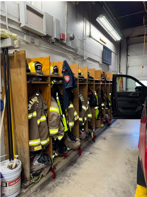
Storage: Clean PPE is stored separately from dirty gear, but this is directly within the apparatus bay, and in plywood (porous material) cubbies that can hold onto contamination.
