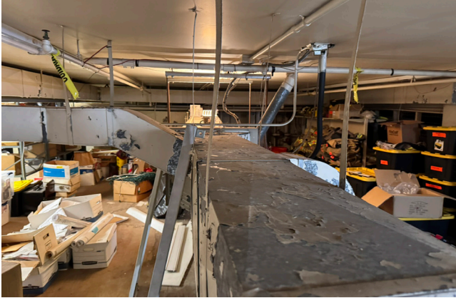
Current HVAC units: Peeling paint on ductwork; Storage of gear and flammable paperwork near gas fired appliances in mechanical equipment mezzanine.
