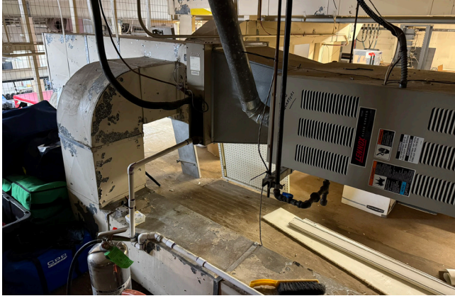
Current HVAC units: Peeling paint on ductwork; Storage of gear and flammable paperwork near gas fired appliances in mechanical equipment mezzanine.
