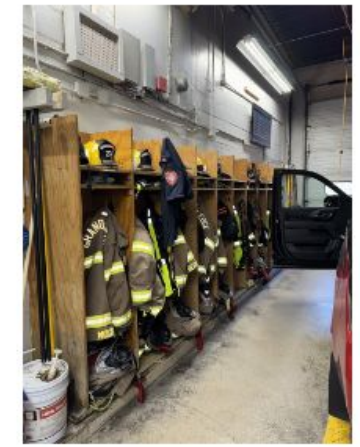
Storage: Clean PPE is stored separately from dirty gear, but this again is directly within the apparatus bay, and in plywood (porous material) cubbies that can hold onto contamination.
